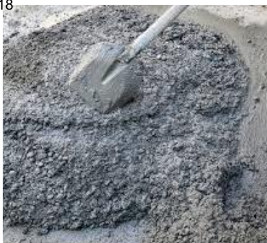
Mixing of concrete
